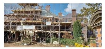
In August 2019 Betley Court suffered a devastating fire which destroyed much of the property, including almost all of the interior and roof structure. This is presently being reinstated and much of this structural and enveloping work is complete and the scaffolding is incrementally being removed.
